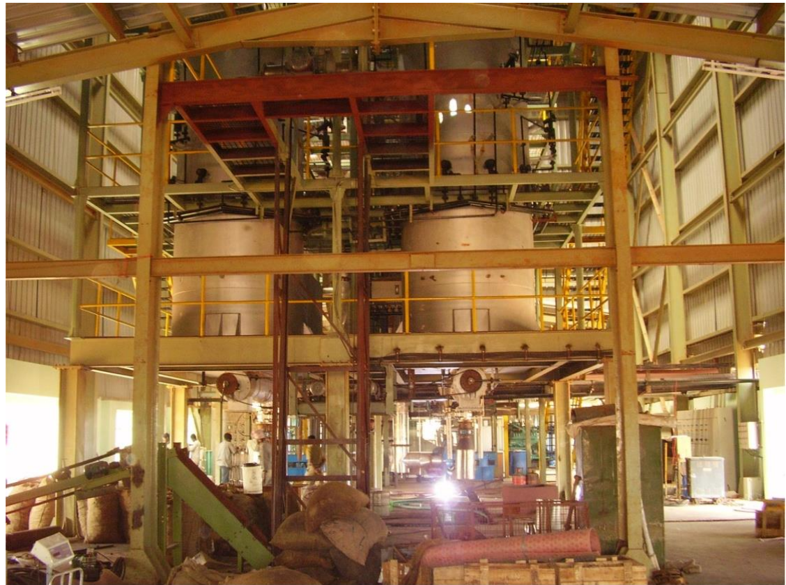
BMC GASIFIER PLANT(1700Kgph)
